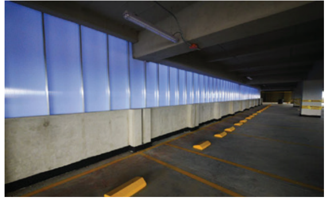
Car parking structures
